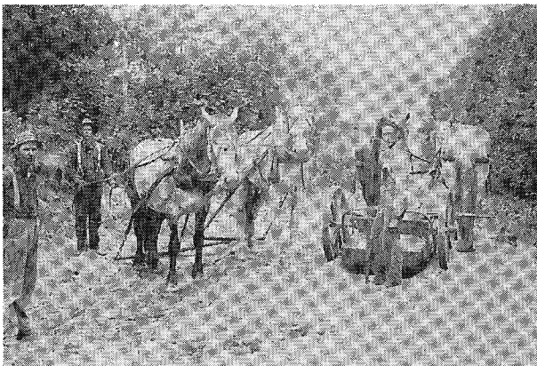
A Township road crew prepares 604, west of Butwell Road, for planking.
